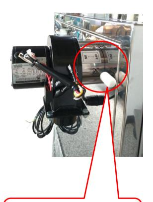
**Step 1:** Flip off the exhaust damper
